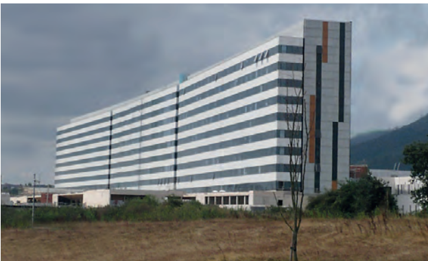
Hospital Central, Asturias
